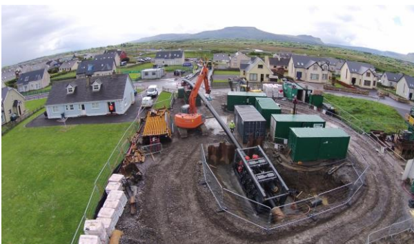
Pipe installation overview with Pipe Pusher in position
