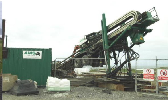
Prime PD250 Drill Rig in position
