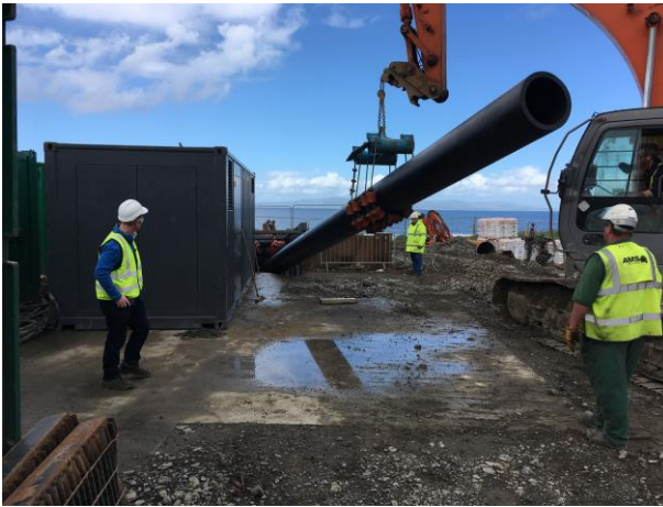
Pipe Installation Complete
